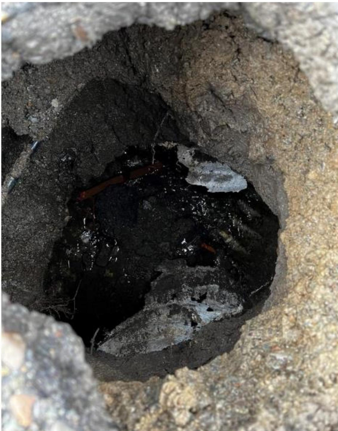
Figure 2: Photo taken inside the sinkhole located at the intersection of Conklin Road and Ridgemont Drive. Soils have eroded and top of culvert has rusted and collapsed. Photo taken 12/27/2023.
