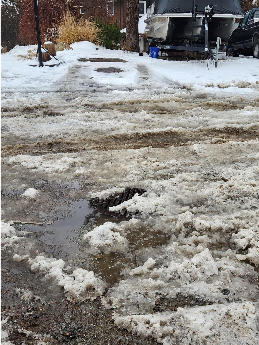
Figure 24: Failing drywell observed in Cameron Court cul-de-sac by Osborn. Photo taken 1/22/2024.
