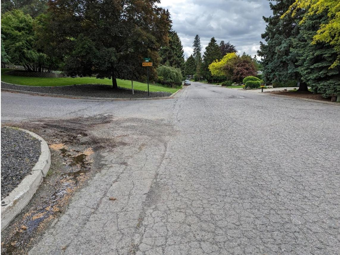
**Figure 3-6. Roadway failure observed at South Vera Crest Drive and East 20th Court**
