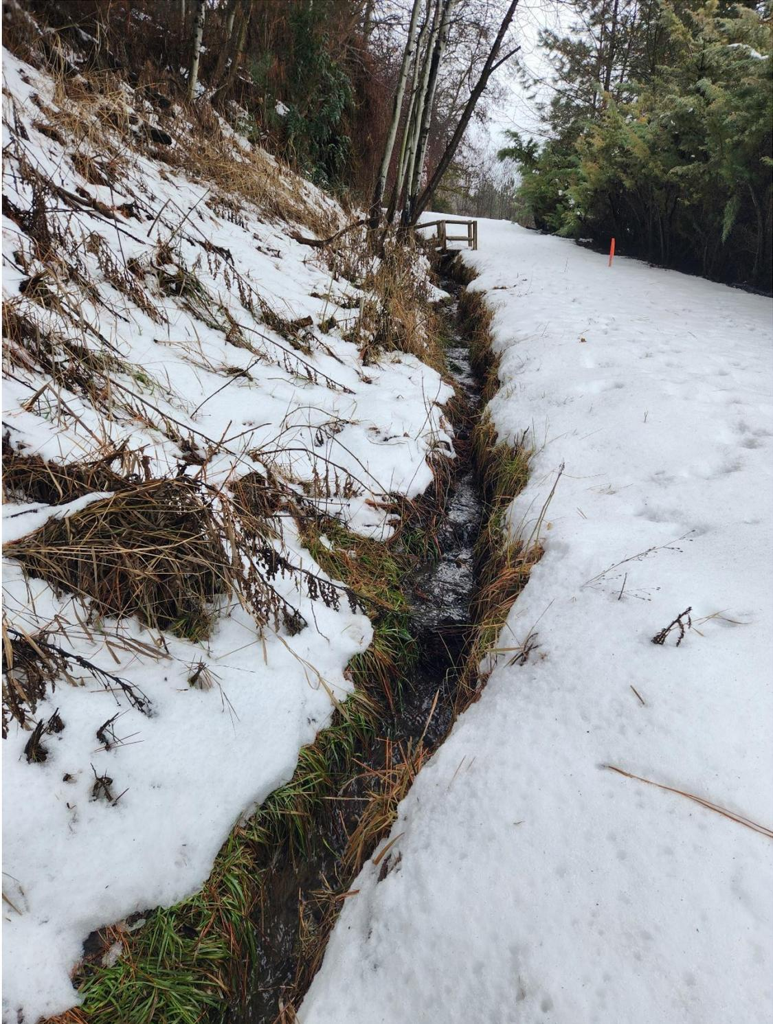
Figure 7: Upstream end of the Radco open channel ditch. Flow is clearly visible in the open channel, but seems to dissipate the further down the open channel you go. Photo taken 1/22/2024.
