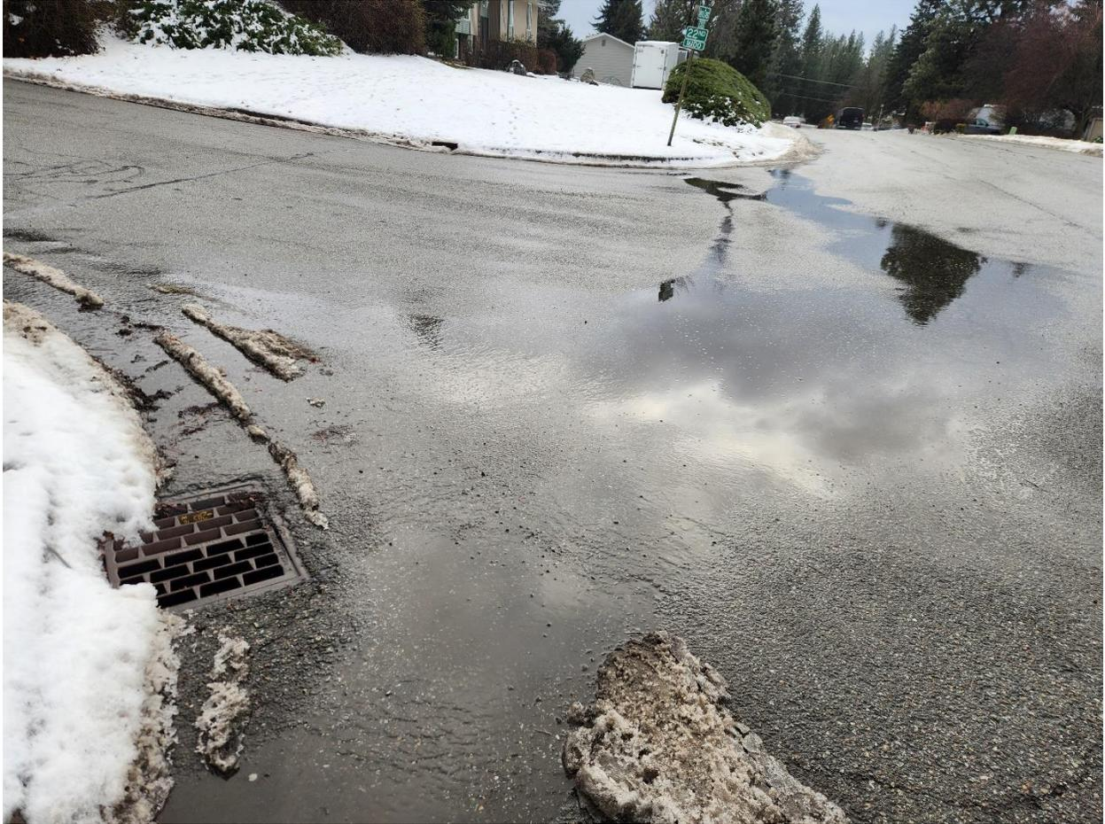
Figure 15: Ponding water at the intersection of 22nd Avenue and Vera Crest Drive. Water has been observed to pond here during various site visits, failing to reach the catch basin shown in the picture. Photo taken 1/22/2024.
