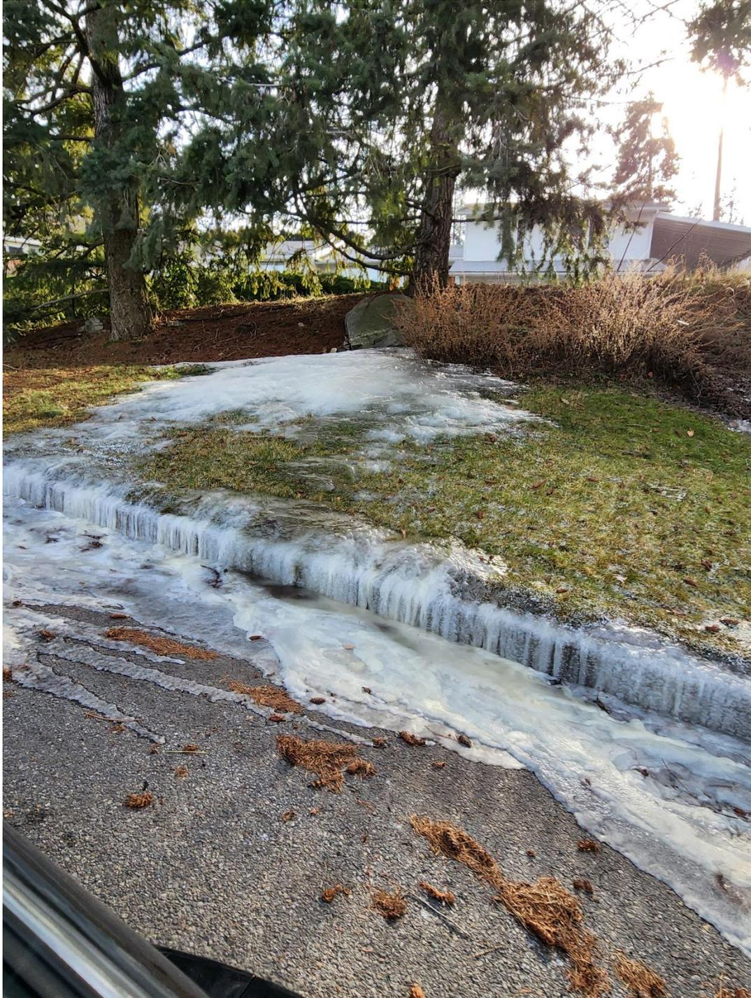
Figure 17: Qalert submitted by resident with groundwater springs on 24th Avenue 6/3/2019. Osborn observed these conditions in the field and took this picture during abnormally cold weather. Photo taken 1/16/2024.
