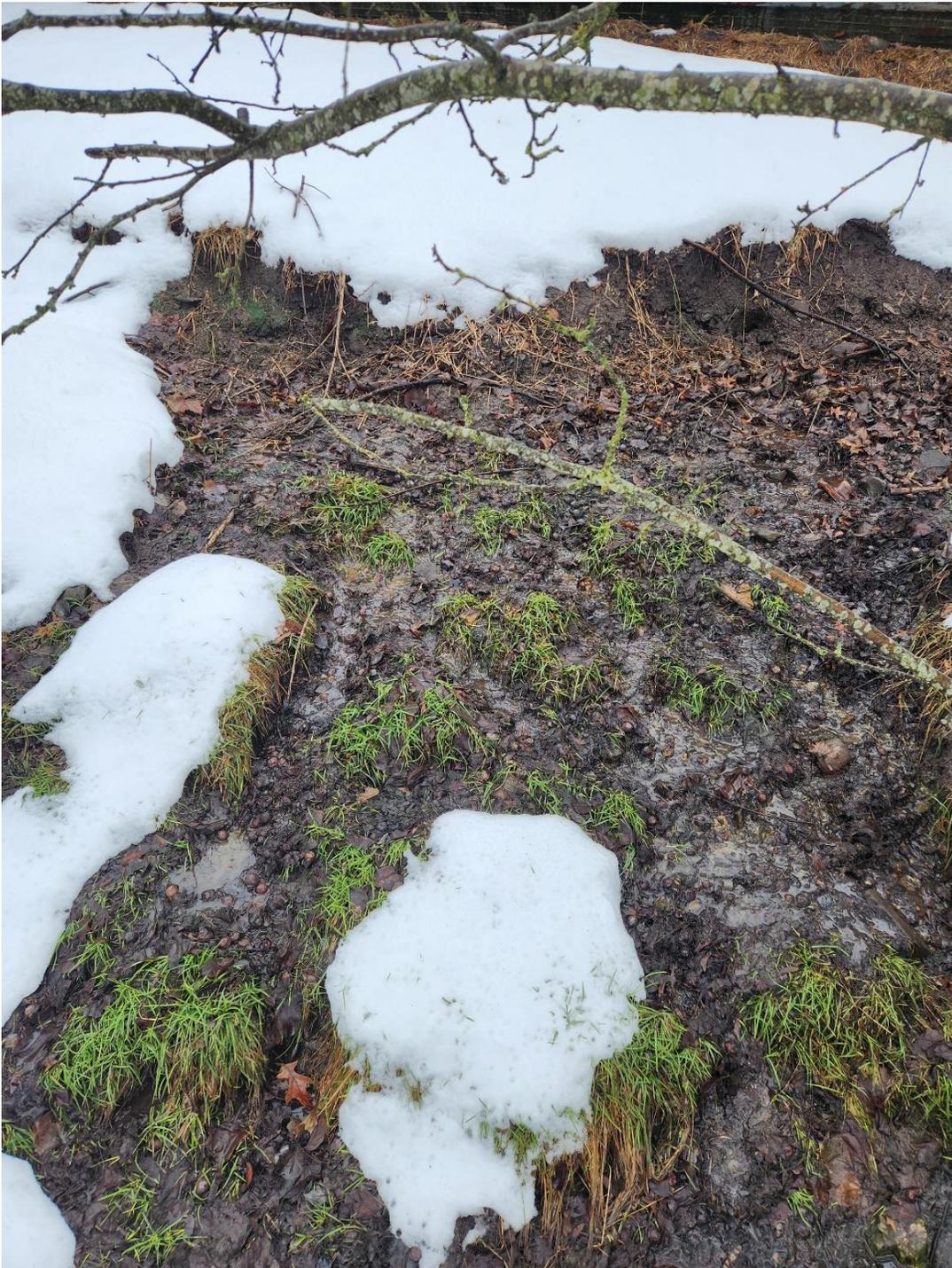
Figure 6: Ground water seeping out of hillside at the top of the Radco open channel ditch. Observed by Osborn in the field during wet conditions. The pipe which runs down this hillside is 50% collapsed and is likely infiltrates water into hillside. Photo taken 1/22/2024.
