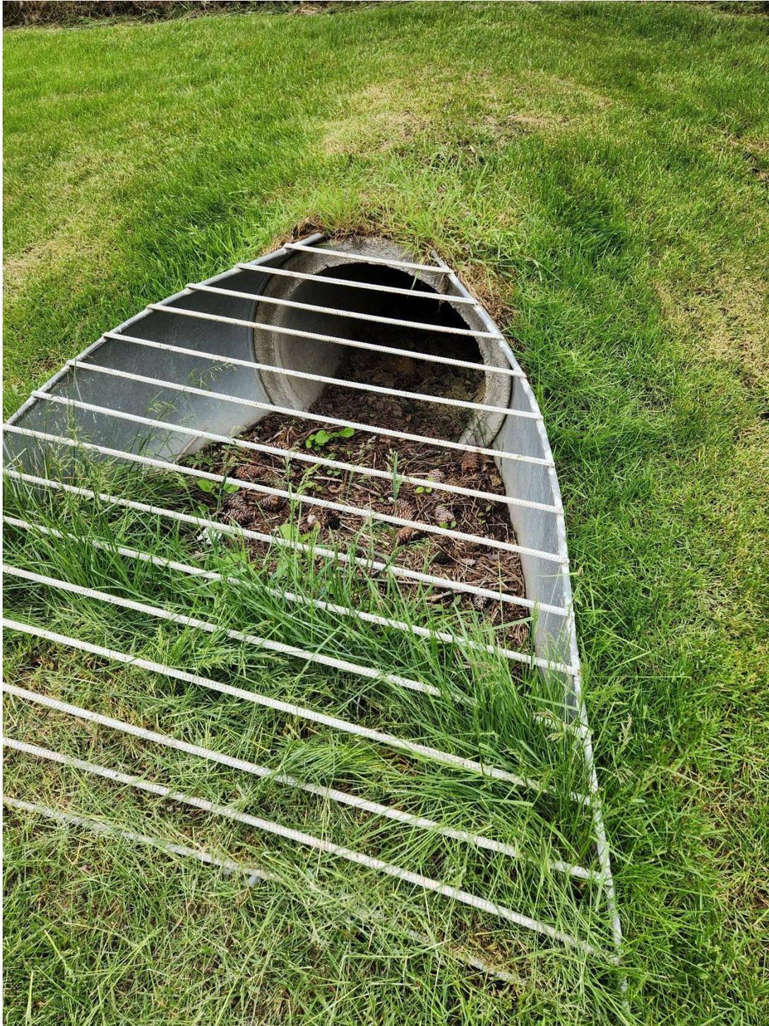
Figure 12: Outlet pipe to the Radco infiltration pond intended to convey flow from the Radco open channel ditch. Pipe observed to be dry throughout various site visits, reinforcing the belief that water is not reaching this pond. Photo taken 5/28/2024.
