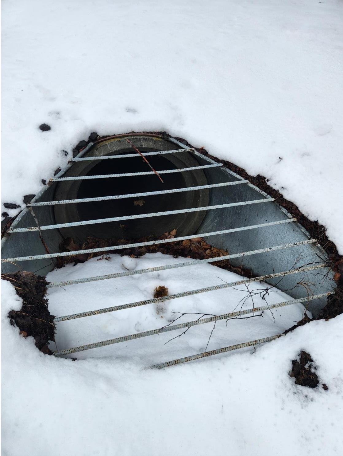
Figure 10: Inlet pipe located at the end of the Radco open channel ditch. Despite flow being present higher up in this open channel ditch, flow does not reach this inlet pipe and has been observed to be dry. Photo taken 1/22/2024.
