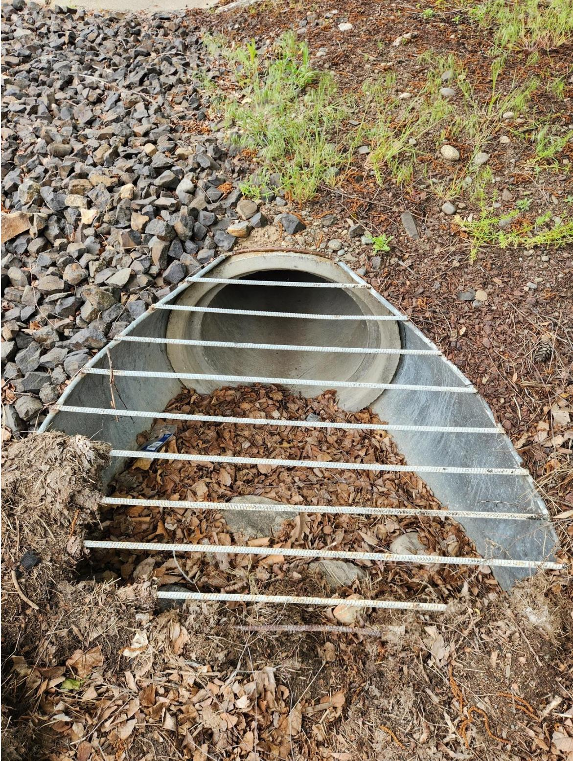
Figure 11: Inlet pipe located at the end of the Radco open channel ditch. Photo taken 11/16/2024.
