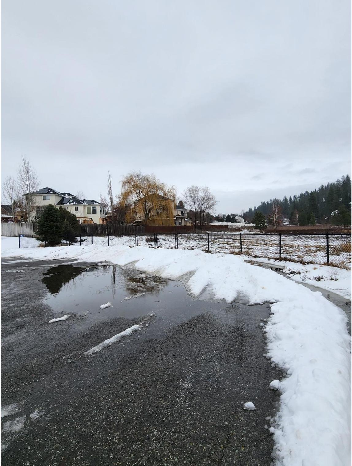
Figure 3: Ponding water at the Radco Drive cul-de-sac. Heavy ponding with nowhere for the water to drain causing damage to the road. Photo taken 1/22/2024.
