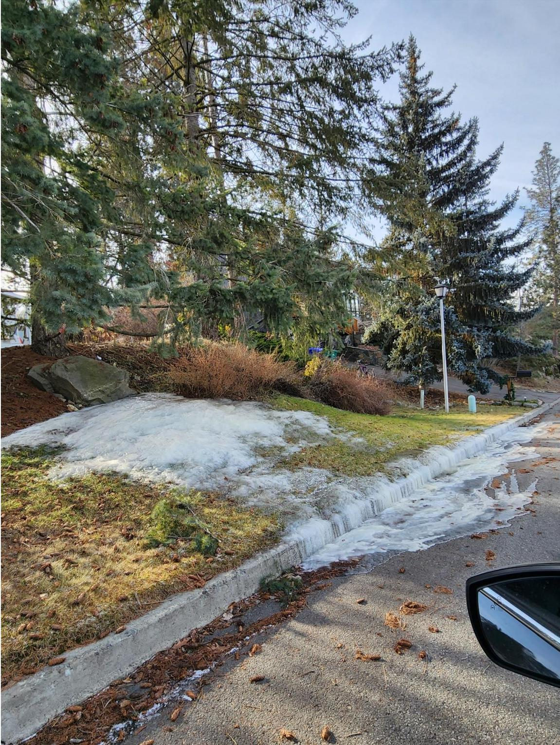
Figure 18: Qalert submitted by resident with groundwater springs on 24th Avenue 6/3/2019. Osborn observed these conditions in the field and took this picture during abnormally cold weather. Photo taken 1/16/2024.
