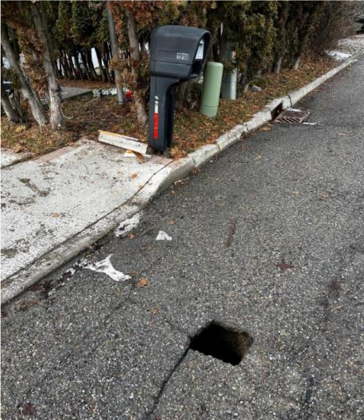
Figure 1: Sinkhole at the intersection of Conklin Road and Ridgemont Drive observed by city maintenance crew and submitted as a QAlert 12/27/2023. Photo taken by maintenance crew; hole was then covered by large metal plate.
