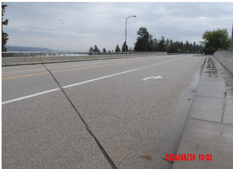
Mission Avenue over Evergreen bridge with new deck overlay and new compression seals, SPOKV-4518.
