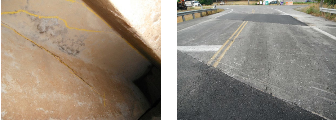
Shear crack at north end of Girder C, east side, and reflective cracking in the bridge deck, SPOKV-4520
